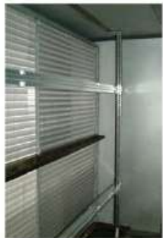
Fig. 8 Horizontal Lamp Placement for Coil Surface Disinfection
